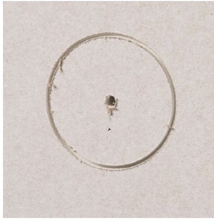
Do not drill the first hole completely.
