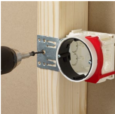
Fastening with one gypsum screw.
