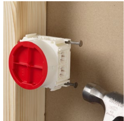
Also possible to fasten with nails.
