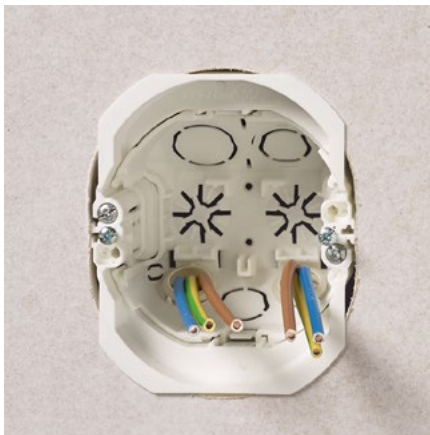
Flexible plastic conduits are attached and the box is fully installed in the hole.
