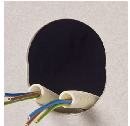
Pull out the flexible plastic conduits from the hole.
