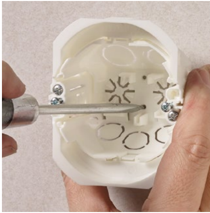
Drilling template is marked on the bottom of the box.
