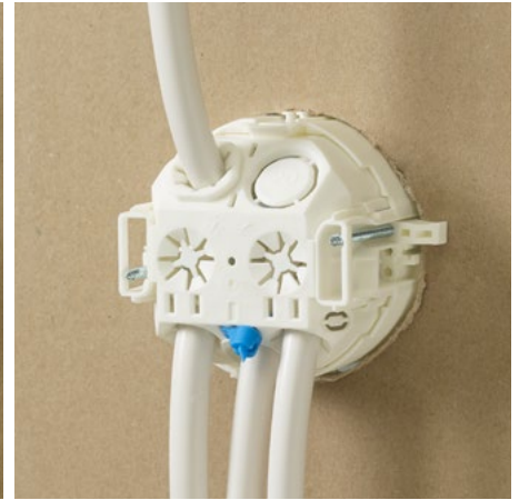
Flexible plastic inlet can be used for cable installations by using cable ties as cable clamps.
